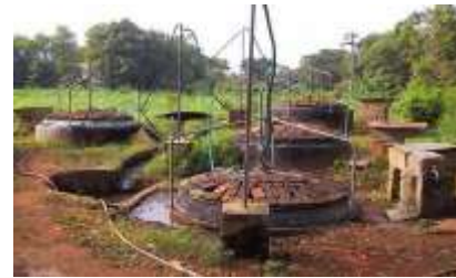
Gambar 4 Proses Penimbunan Digester ,Bak Control,Lubang Inlet,Lubang Outlet
