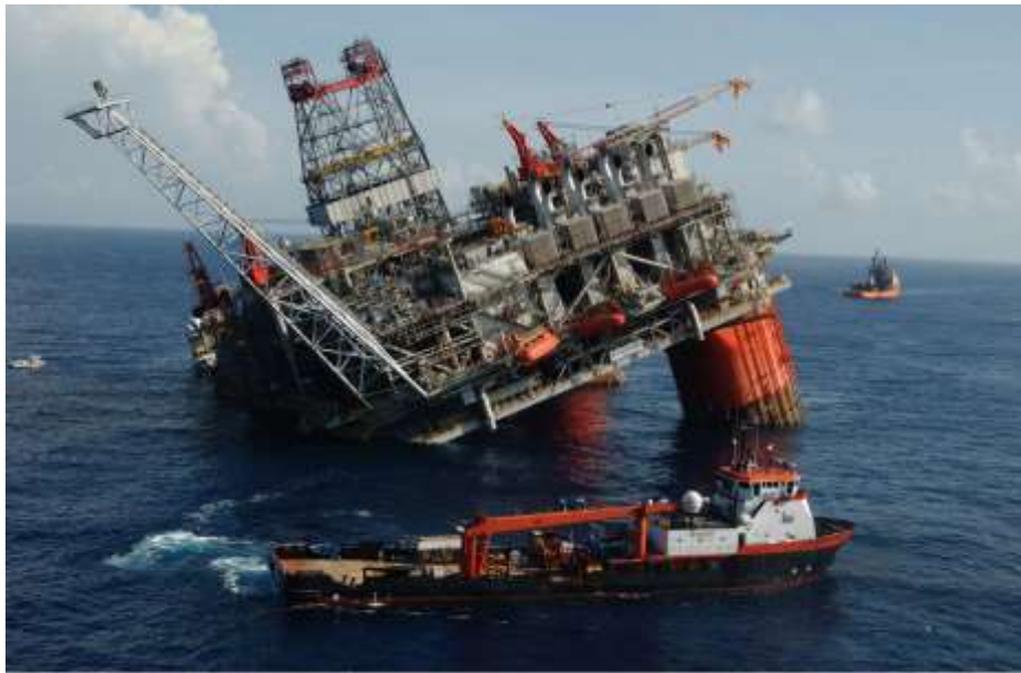
Figure 1. BP's Thunder Horse Platform Listing after Hurricane Dennis
